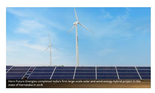
1st HFE's wind- solar hybrid project is at Kavithal district, Karnataka, India. In an existing 50MW wind farm, we added another 28.8MW solar PV site to form this pioneering hybrid system, to cater to clean energy requirements of corporations in that state, thereby offering better grid infrastructure utilization and a step towards making renewable behave like a base load.
